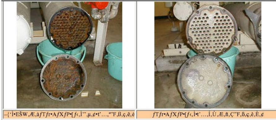
**Compressor Heat Exchange Tubes in Japan before and after installation of EcoBeam XL**
